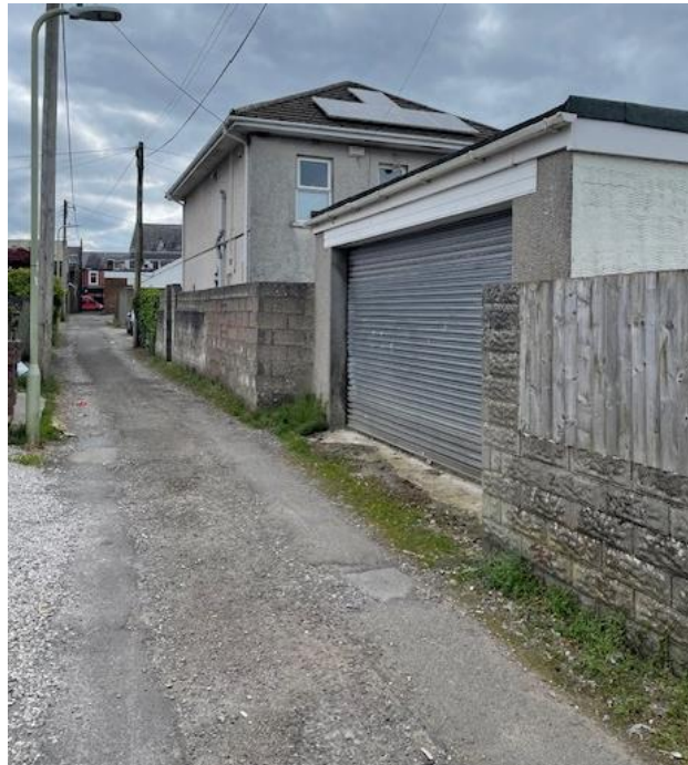
APPLICATION PROPERTY AND GARAGE – LOOKING EAST
